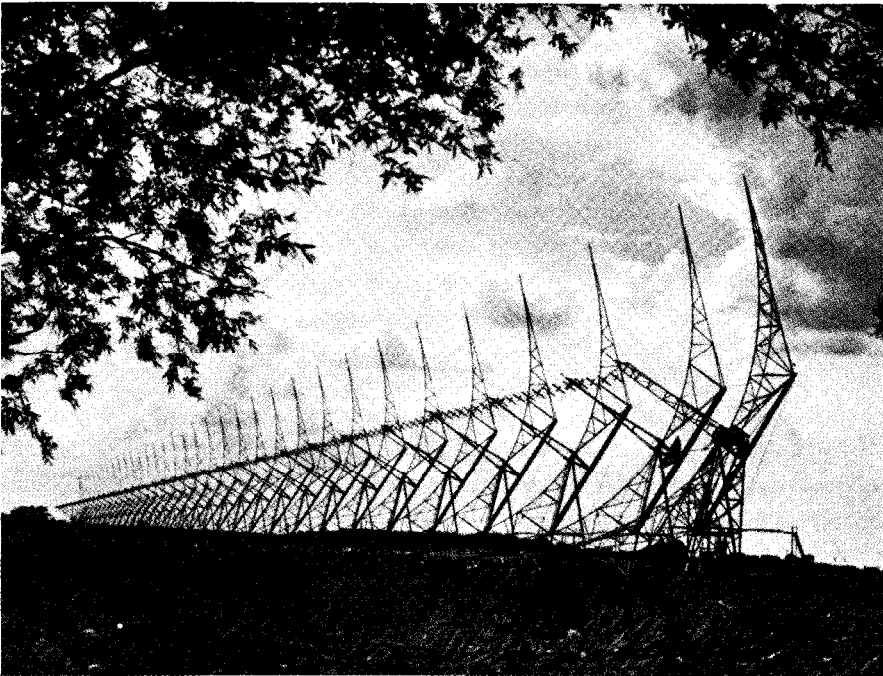
Fig. 3. Photograph of the east-west arm of the \lambda = 1.7 m instrument built in 1957 with which nearly 5000 sources were located.
